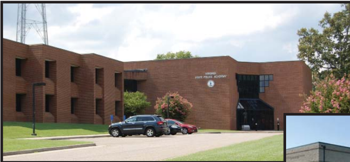
Training Academy, SPHQ Campus, North Chesterfield Campus
